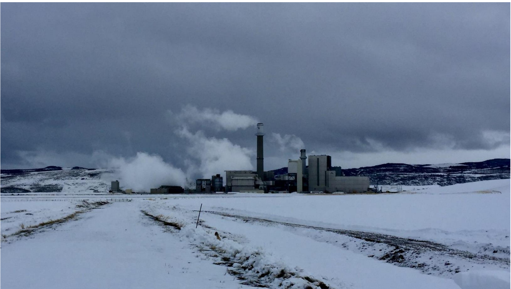
Hayden Generating Station consumed 4.4 million gallons of water each day from the Yampa River
